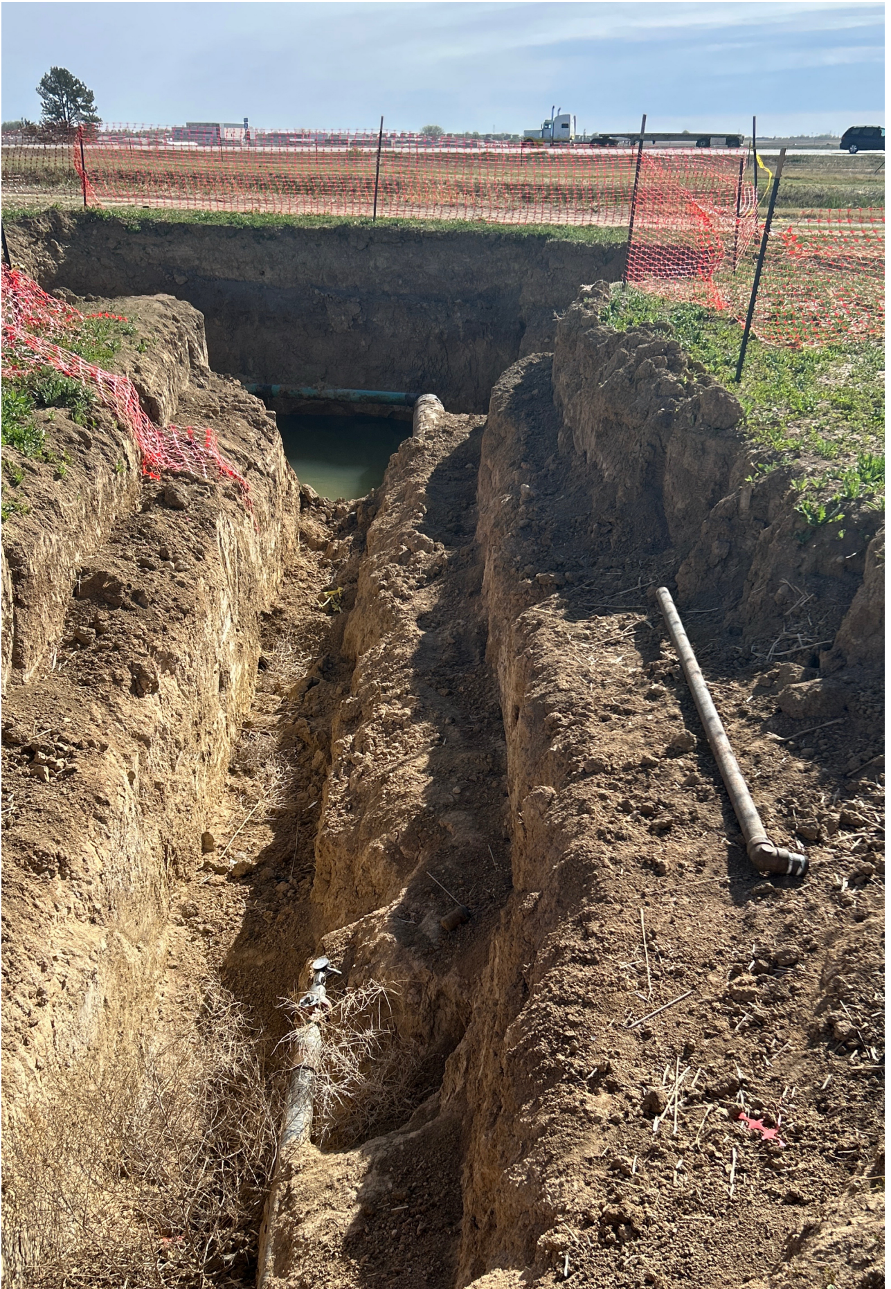
Two flowlines are visible within the excavation.
