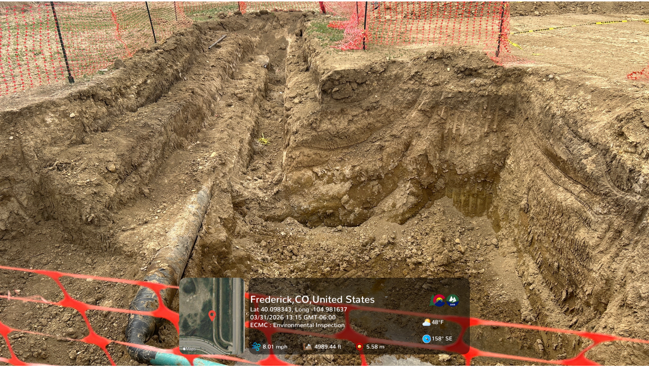
Two flowlines are visible within the excavation.
