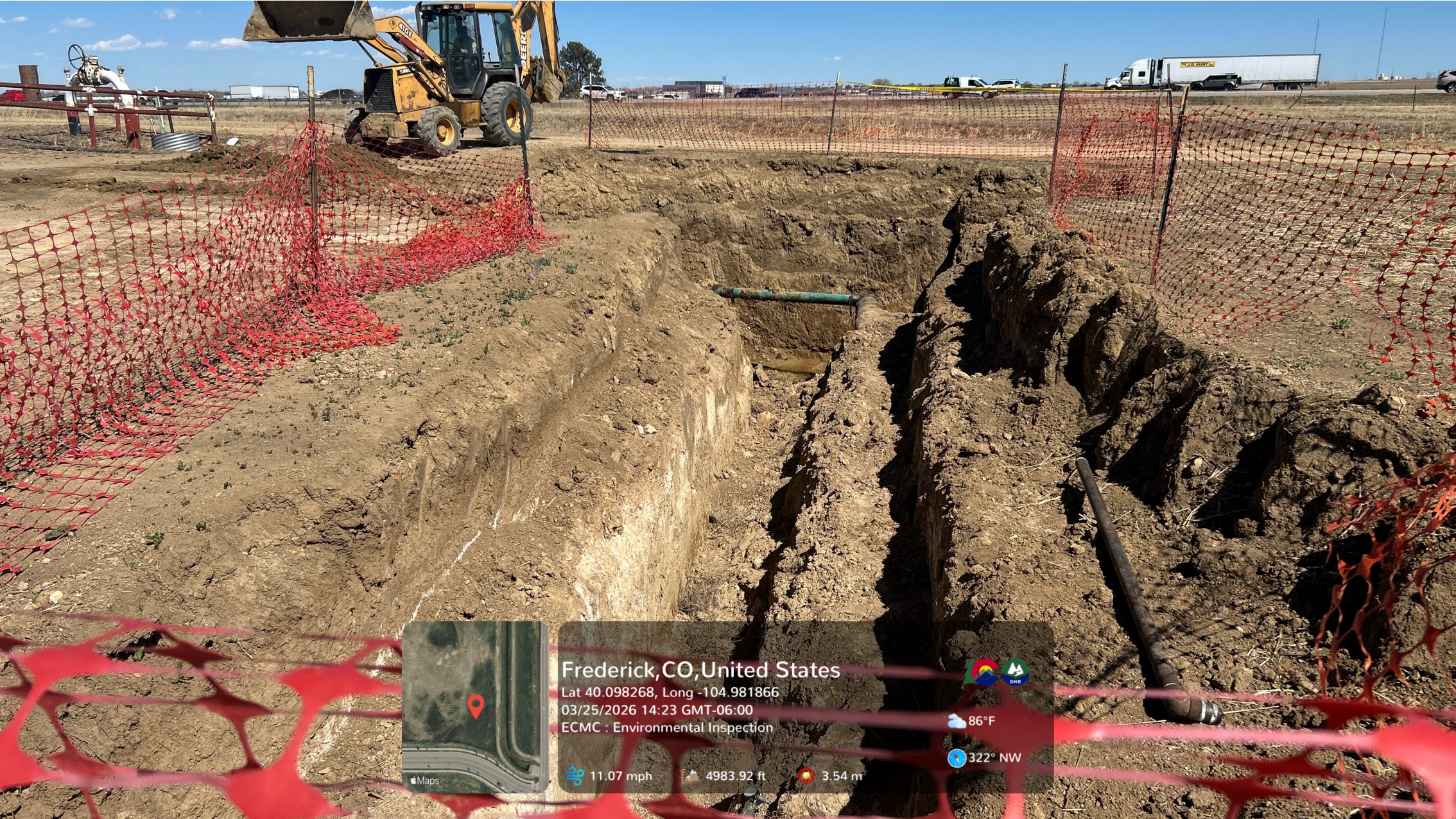
Two flowlines are visible within the excavation.
