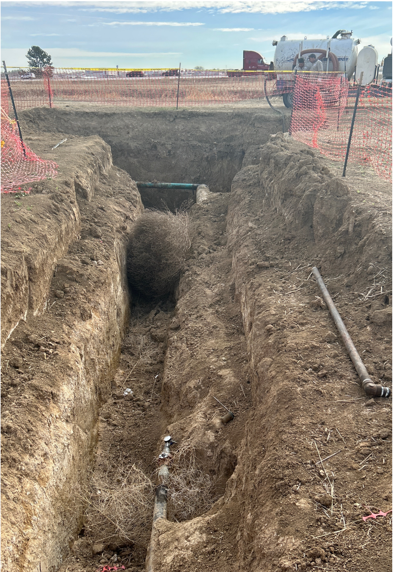
Two flowlines are visible within the excavation.
