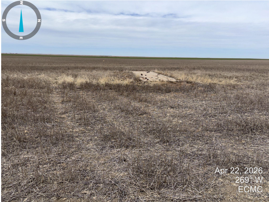
Photo 1. Looking west across the location. A concrete pumpjack pad remains on the location. The location is within a fallow field.
