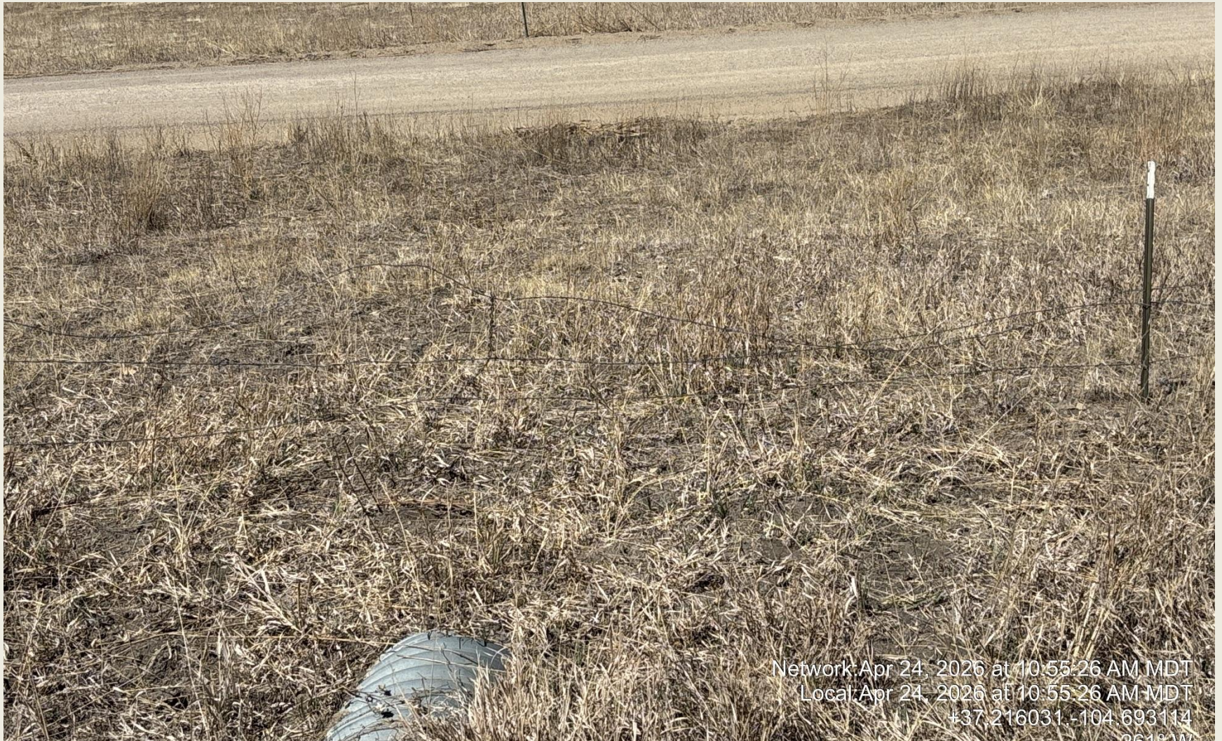
PHOTO 7: DRAINAGE DITCH FROM CULVERT ON ROW TO THE CULVERT THAT CHANELS STORMWATER UNDER COUNTY ROAD IS SILTED IN. CLEAN AND MAINTAIN CULVERT AND DRAINAGE DITCHES PER RULE 1002.f. CA DATE 5/24/2026.
