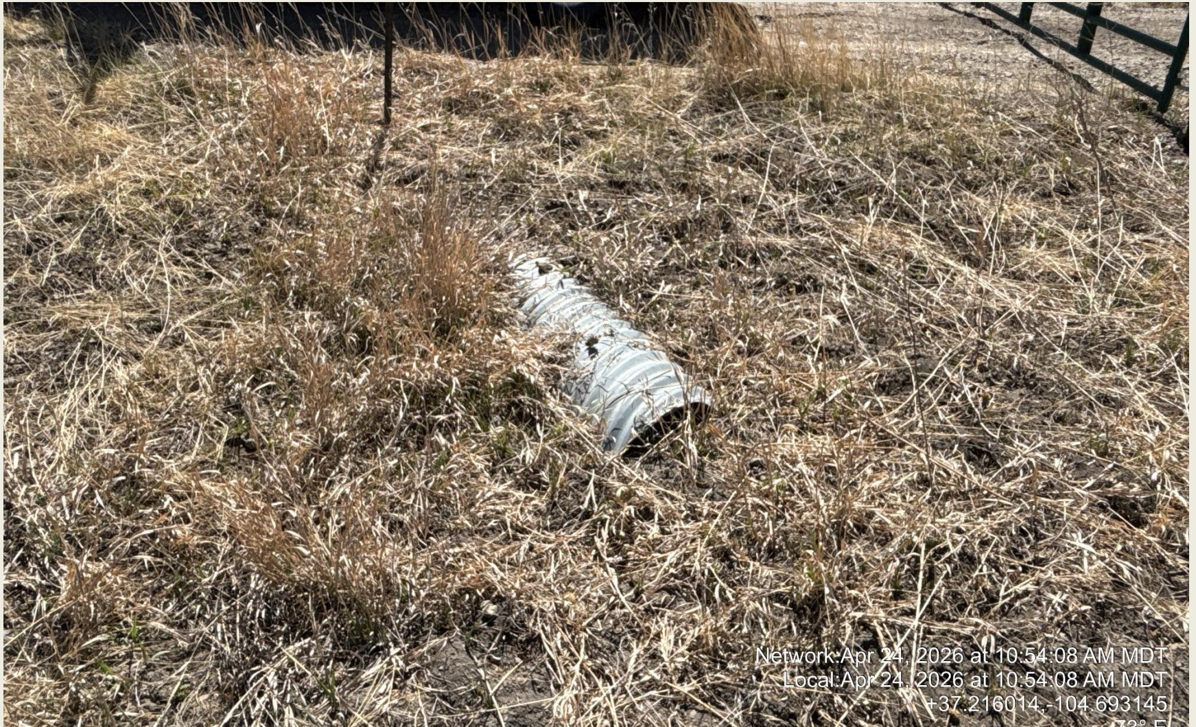
PHOTO 5: CULVERT ON ROW JUST OFF COUNTY ROAD IS PLUGGED. CLEAN AND MAINTAIN CULVERT AND DRAINAGE DITCHES PER RULE 1002.f. CA DATE 5/24/2026.
