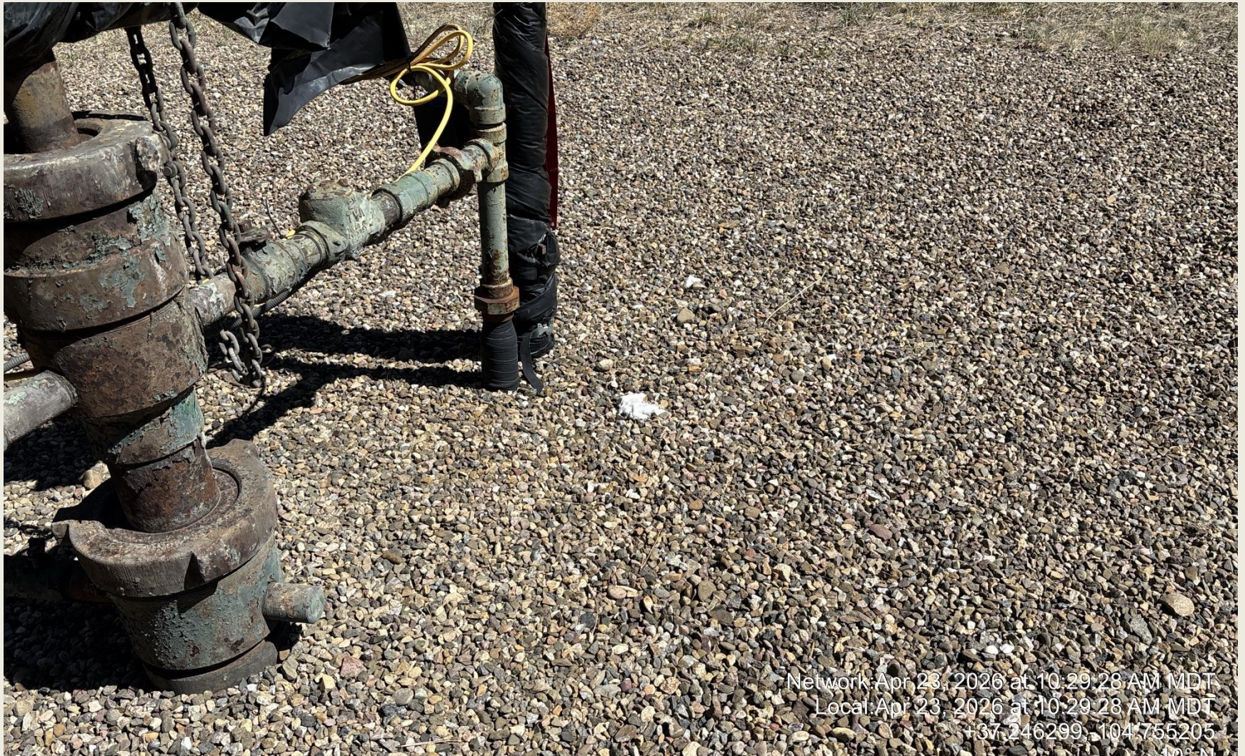
PHOTO 8: MORE IMAGES OF TRASH AROUND LOCATION.
