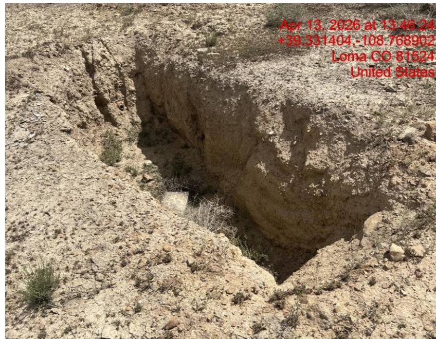
Flowline Excavation – Photo #03521
