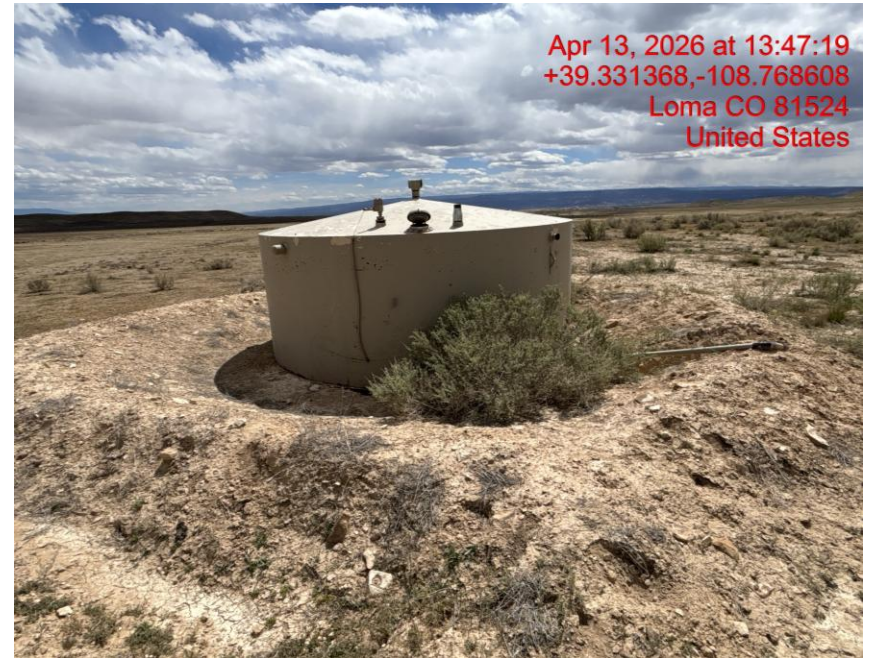
Unused Storage Tank – Photo #03527
