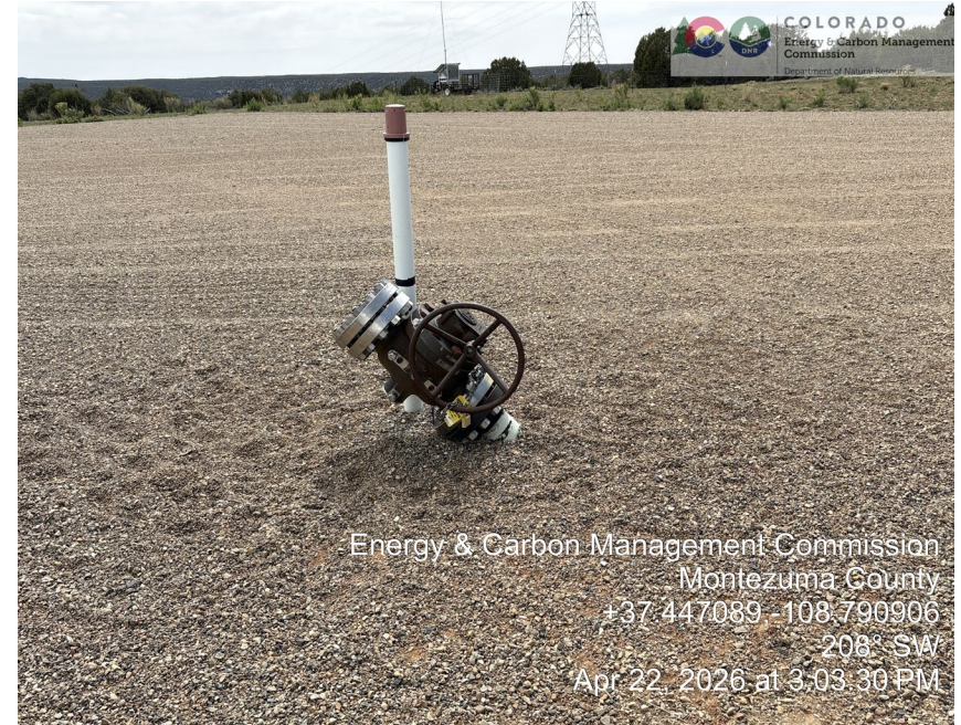
6. Flowline riser disconnected from wellhead. Is marked out of service with yellow tag.
