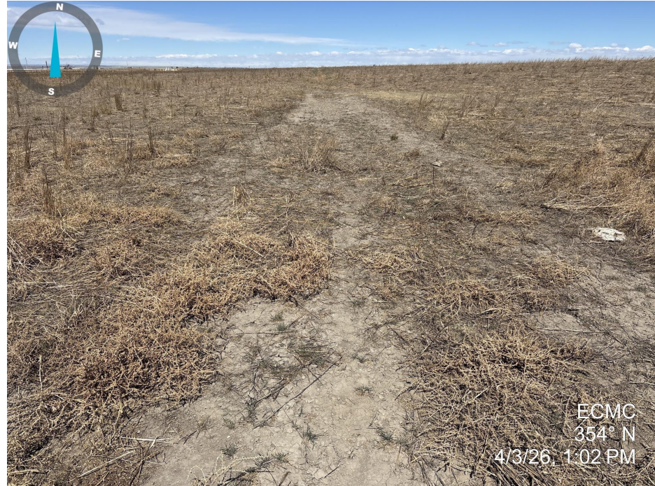
Photo 6. Photo taken of the access road to the well location, facing north. Photo illustrates that the access road does not appear to have been recontoured properly and bare ground and weedy annual vegetation including kochia ( Bassia scoparia ) and russian thistle ( Salsola tragus ) were observed.
