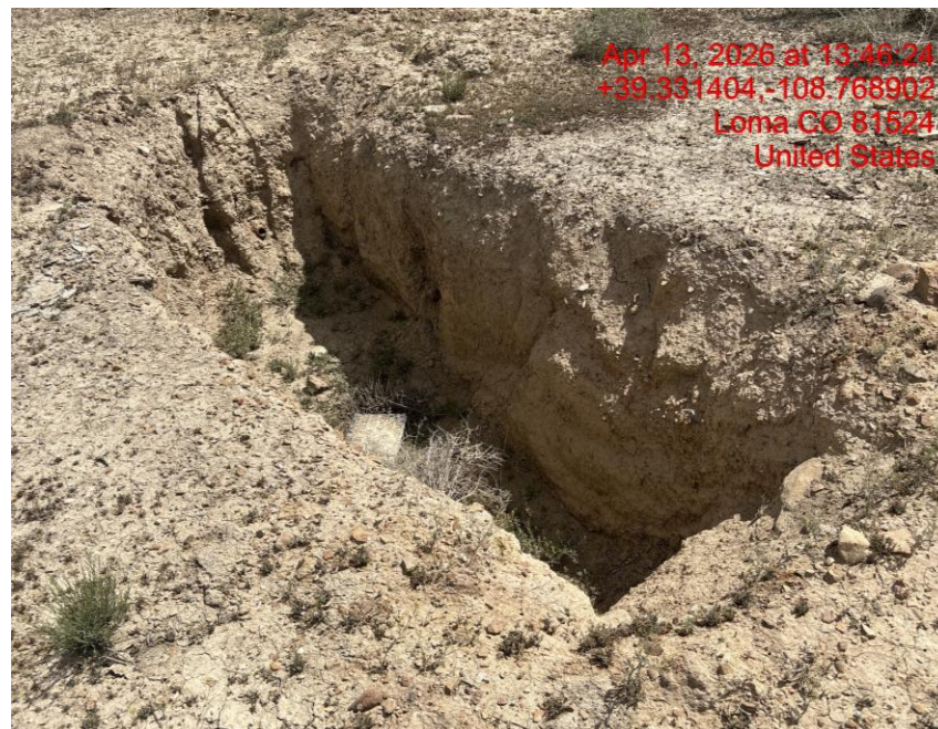
Flowline Excavation – Photo #03521
