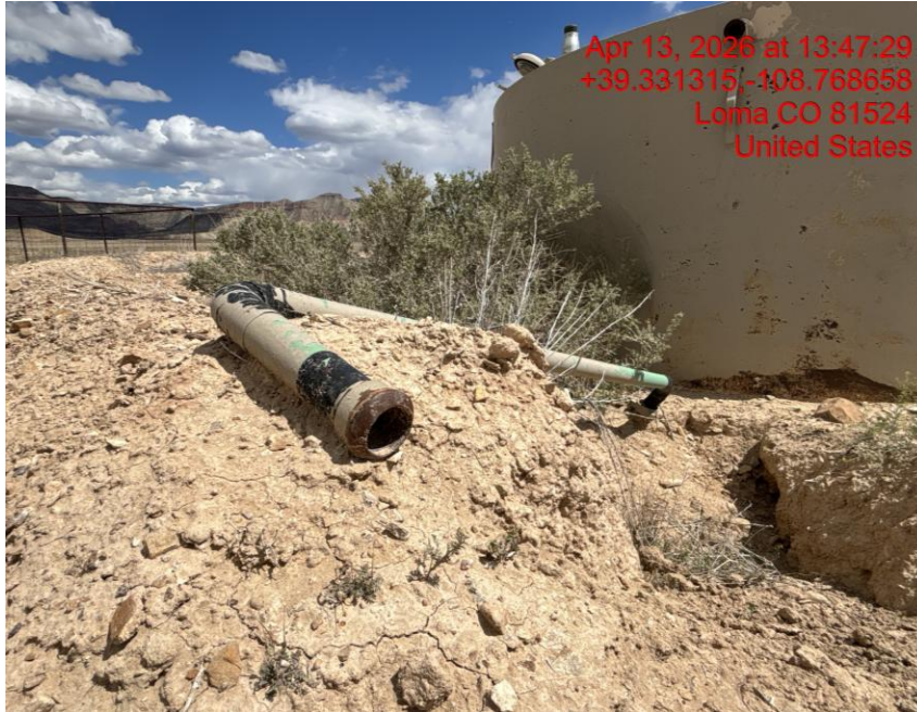
Unused Storage Tank – Photo #03528
