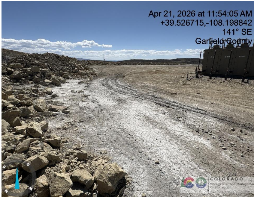
Photo # 1387 Cuttings/E & P waste has migrated onto location/not in compliance with CECMC Rules
