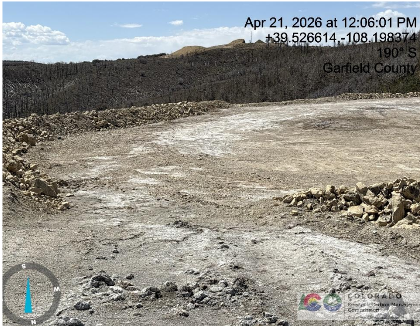
Photo # 1391 Cuttings/E & P waste has migrated onto & across location/not in compliance with CECMC Rules
