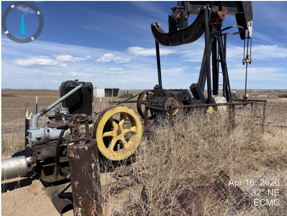
Photo 3. North across the pumpjack. Weeds are in contact with the equipment.
