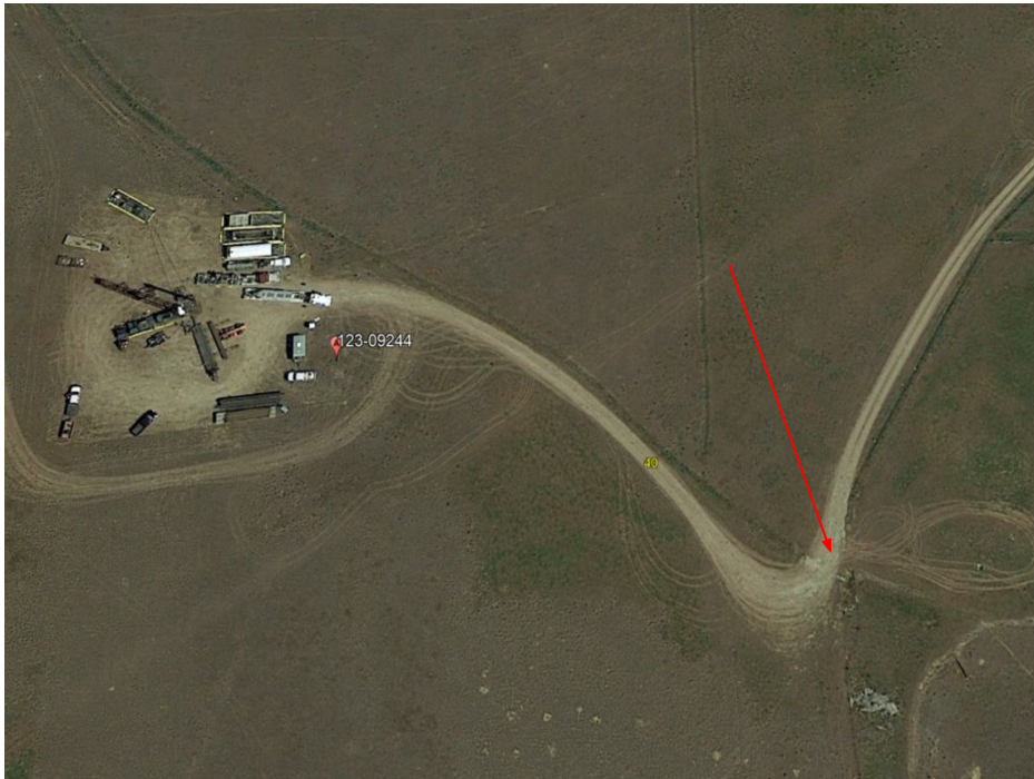
Photo 11. Google earth aerial imagery taken 5/31/2018 while the location was active. A culvert is visible in the access road where it turns and crosses a pre existing ditch.
