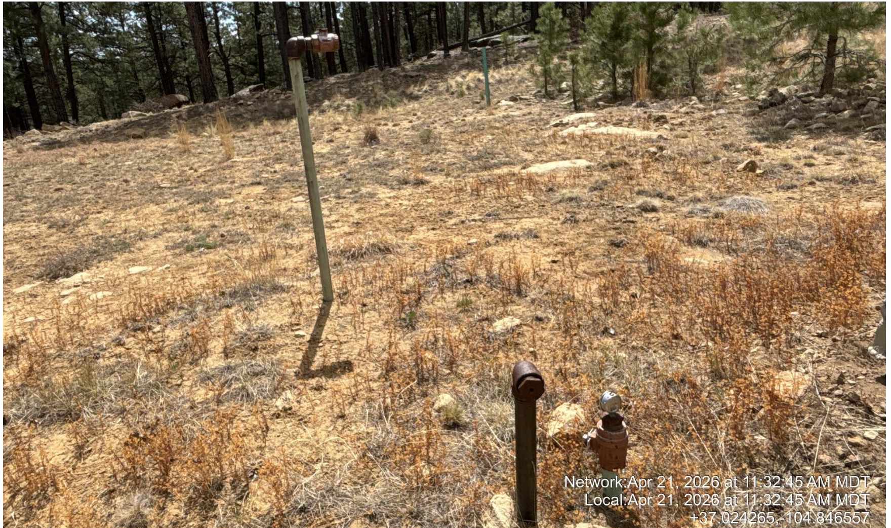
PHOTO 5: UNUSED EQUIPMENT (UNUSED RISERS NEAR WELLHEAD NOT IN USE OR USEFUL). IF RISER ARE NO LONGER USEFUL TO THE OPERATION OF THIS WELL THEY NEED TO BE REMOVED OTHERWISE MARK RISER WITH THERE CONTENTS PER RULE 606. CA DATE 5/21/2026.
