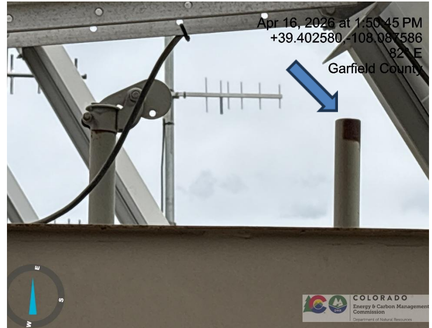
Photo # 148 PRV vent line does not comply with CECMC pressure safety device rules
