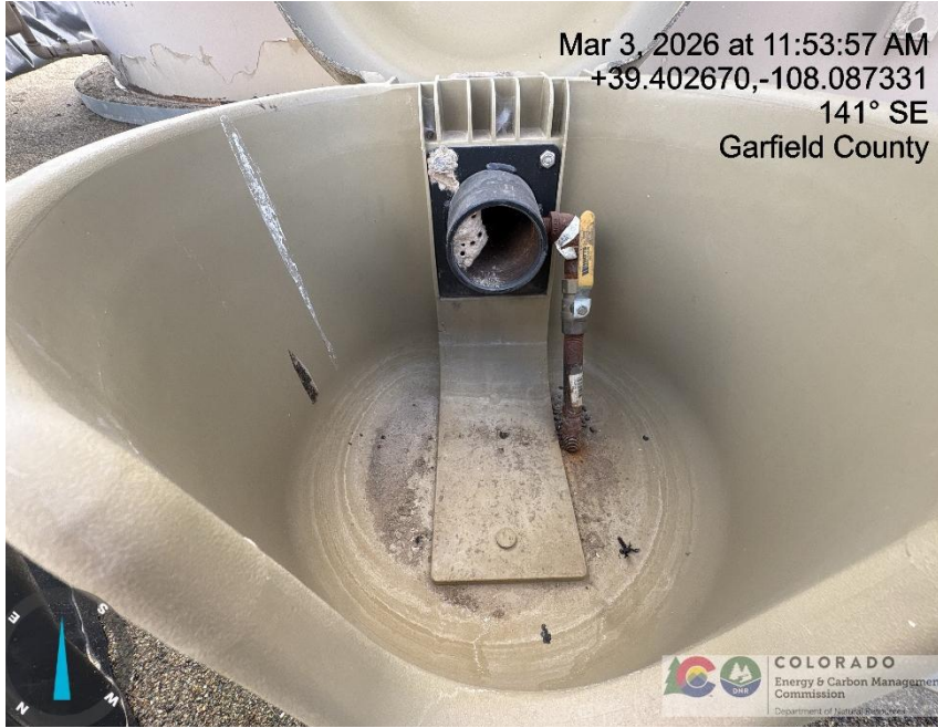
Photo # 4719 From inspection/audit 708908653 conducted on 03/03/2026 - Open ended load line
