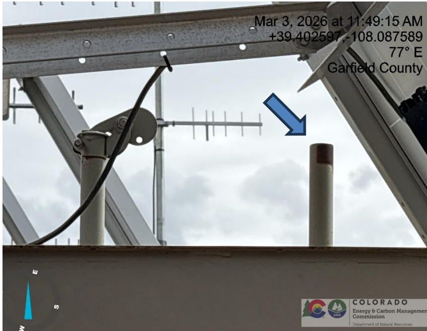
Photo # 4721 From inspection/audit 708908653 conducted on 03/03/2026 - PRV vent line does not comply with CECMC pressure safety device rules
