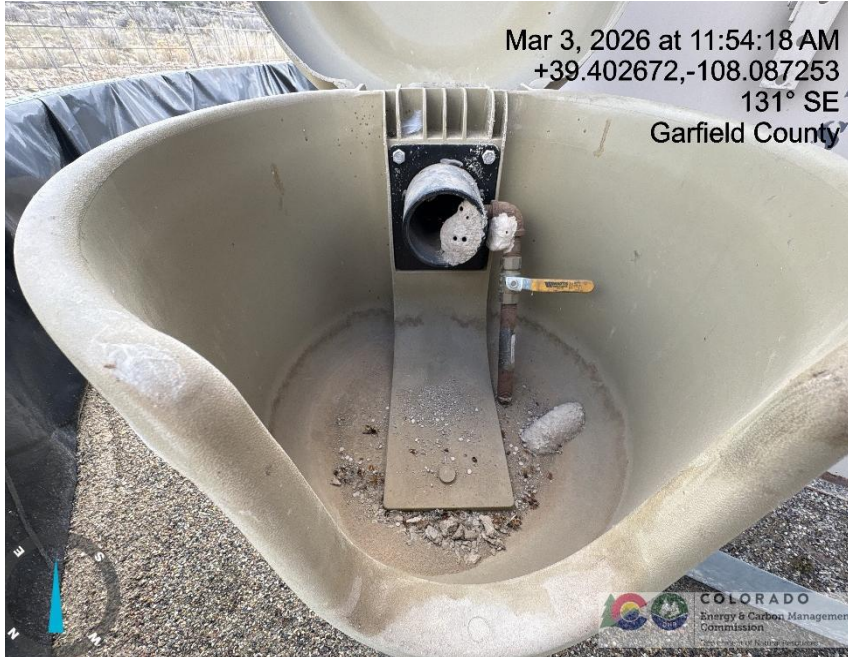
Photo # 4720 From inspection/audit 708908653 conducted on 03/03/2026 - Open ended load line
