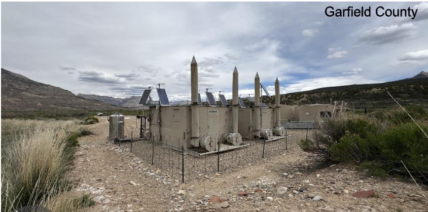
South West corner of location.
