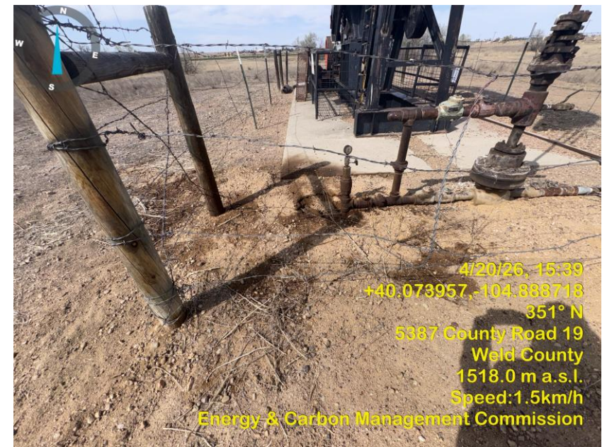
Photo 4 Stained soil by the wellhead.
