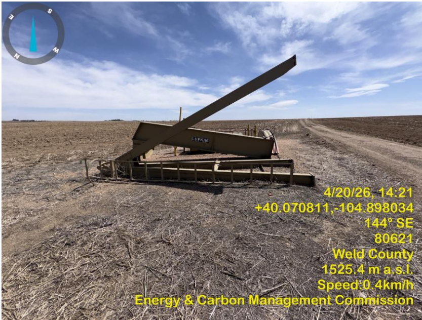
Photo 5 Unused pumping equipment.
