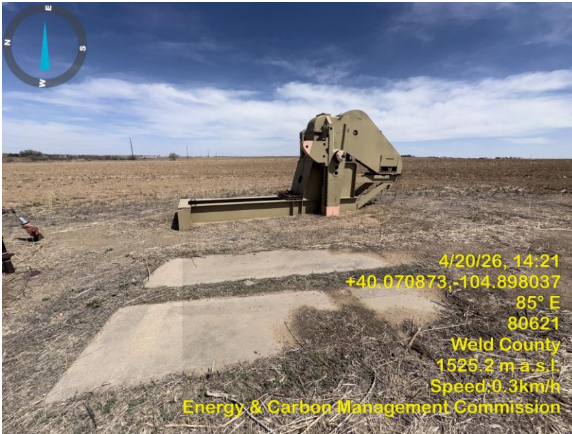
Photo 3 Unused pumping equipment.
