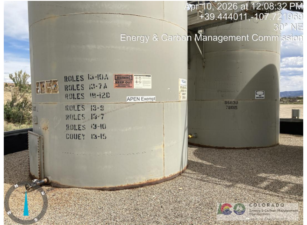
Rust around tank bottoms.
