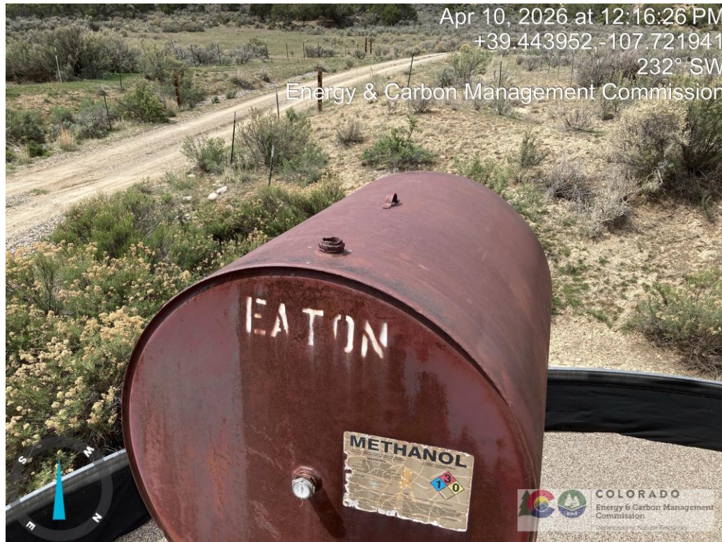
No lid on top of methanol tank.
