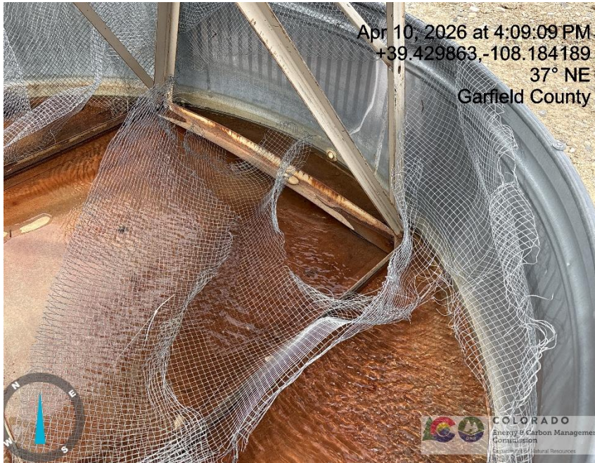
Photo # 8440 Wildlife protection for methanol tank containment needs maintenance
