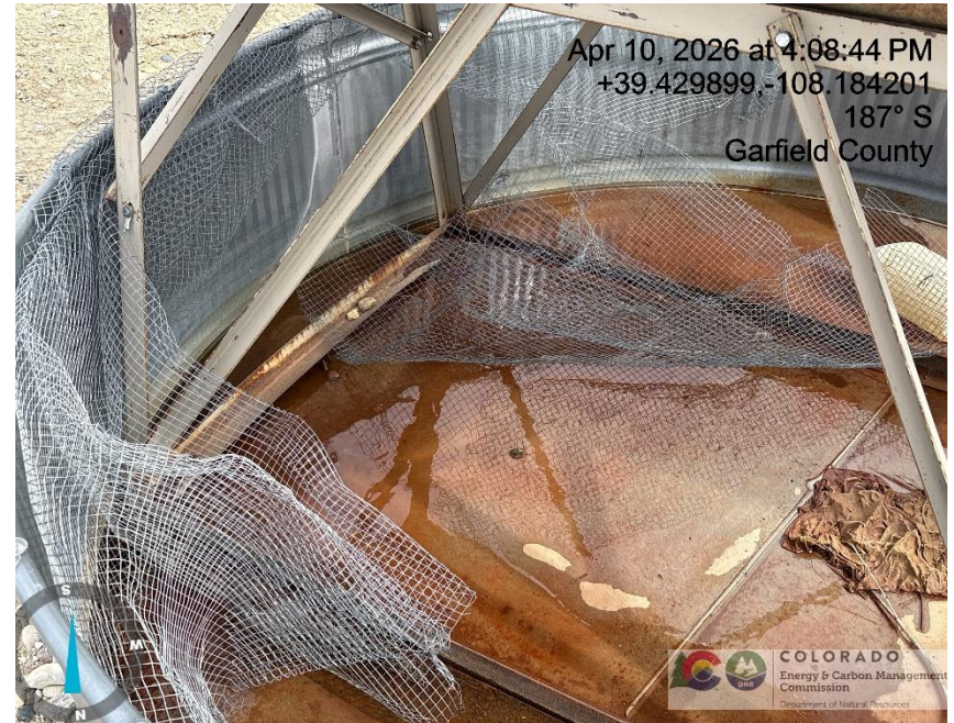
Photo # 8441 Wildlife protection for methanol tank containment needs maintenance
