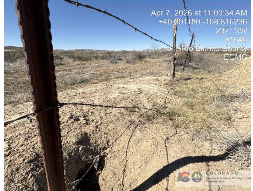
Photo # 4205 Loose barbed wire fencing on location/wildlife hazard
