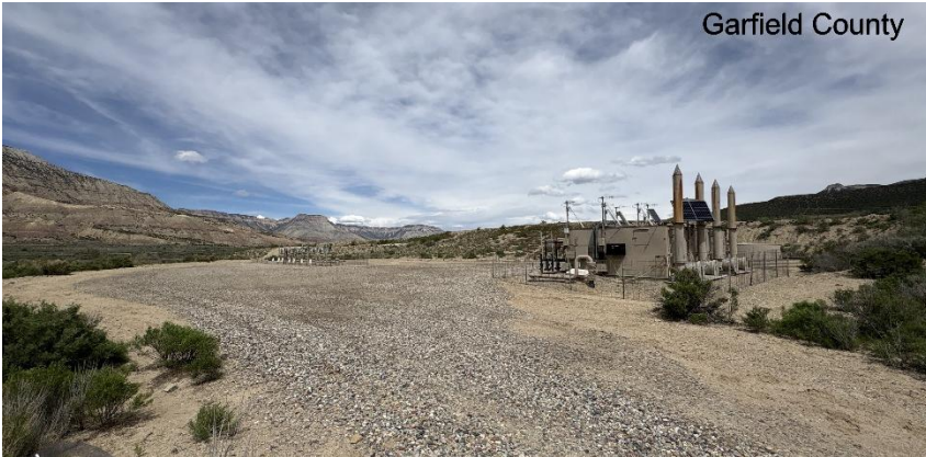
South West corner of location.
