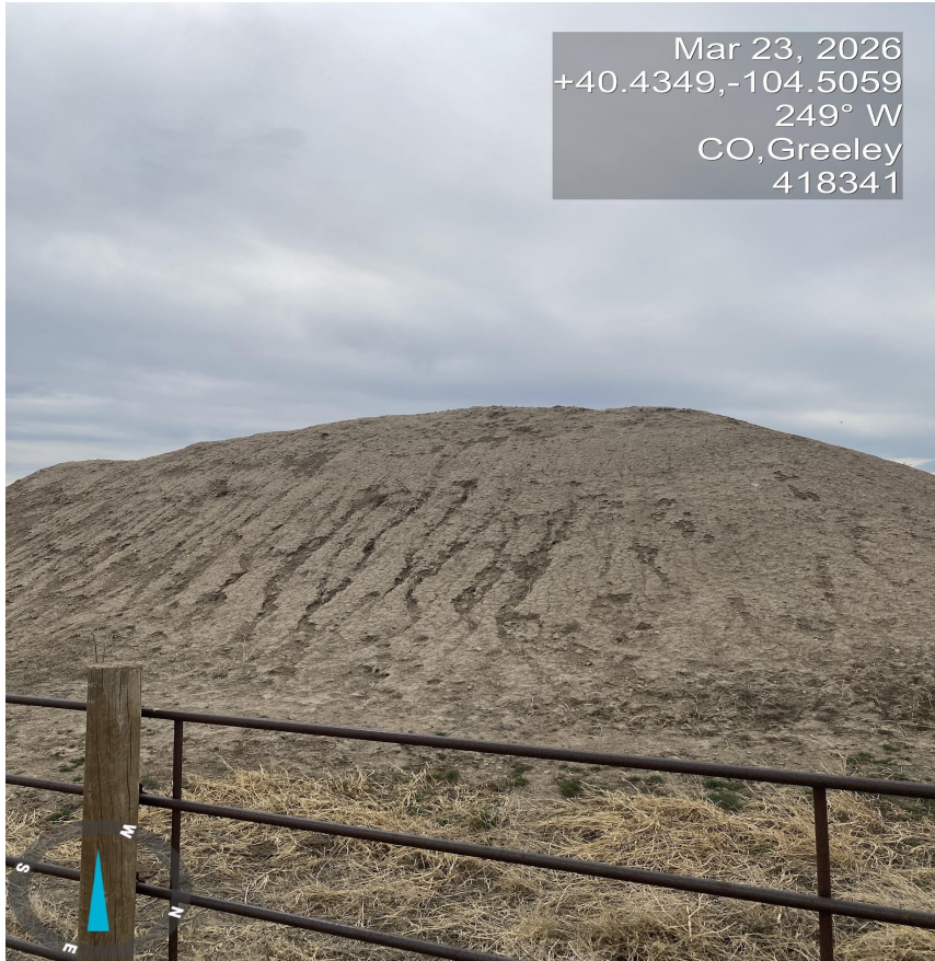
Photo 2. Photo taken of the location topsoil stockpile to the west of the location. Most of the pile is unvegetated and has evidence of rill erosion on it.
