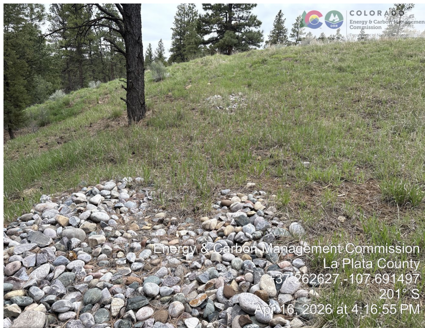
11. Sediment trap and ditch on east side of pad.
