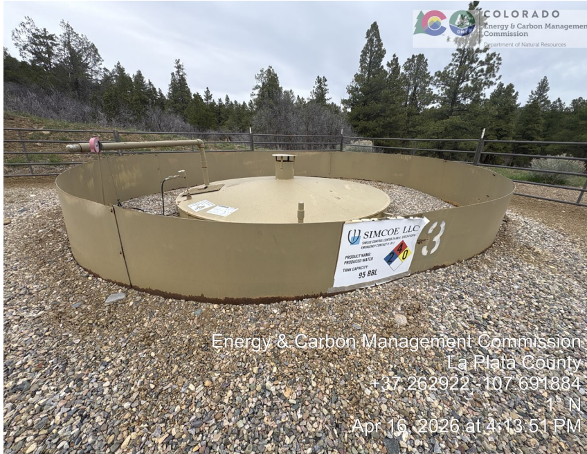
9. 95 BBL PBV steel tank with secondary containment.
