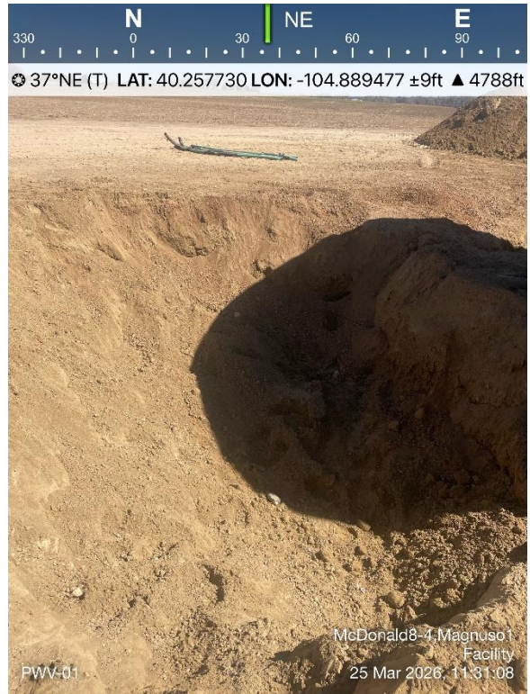
Produced Water Vessel 01 Excavation
