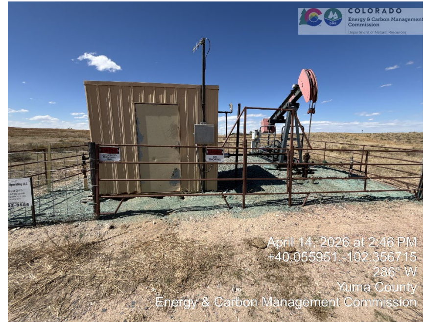
Meter run, Wellhead, and PU
