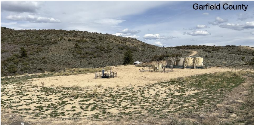
South West corner of location.
