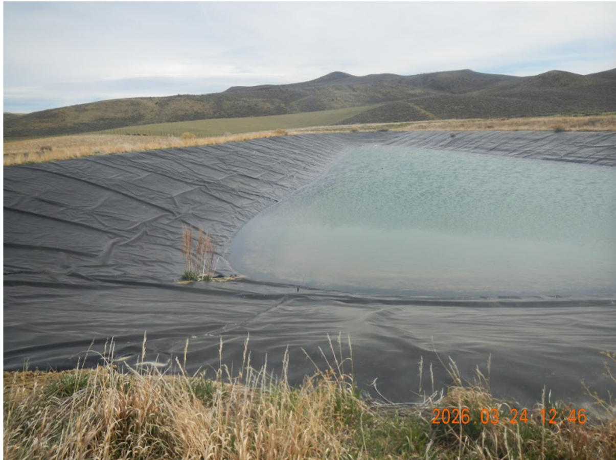
Photo 10 - Pit 2 looking east. Depth of fluids is approximately 12" to 24".
