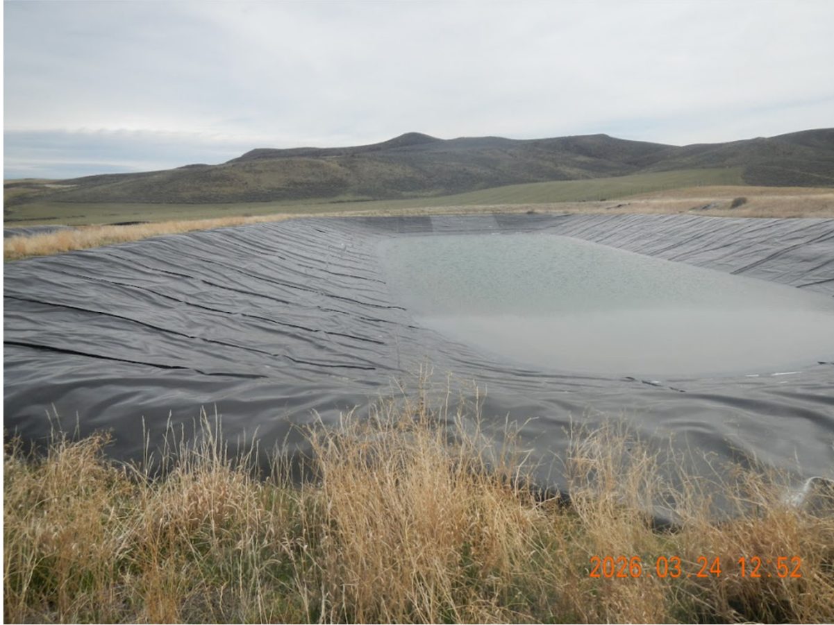
Photo 22 - Pit 6 looking East.. Depth of fluids is approximately 12" to 24".
