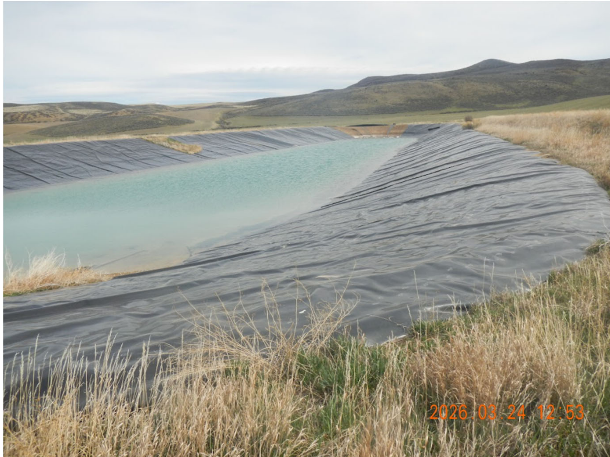
Photo 25 - Pit 7 looking East. Liner is in disrepair. Depth of fluids is approximately 12" to 24".
