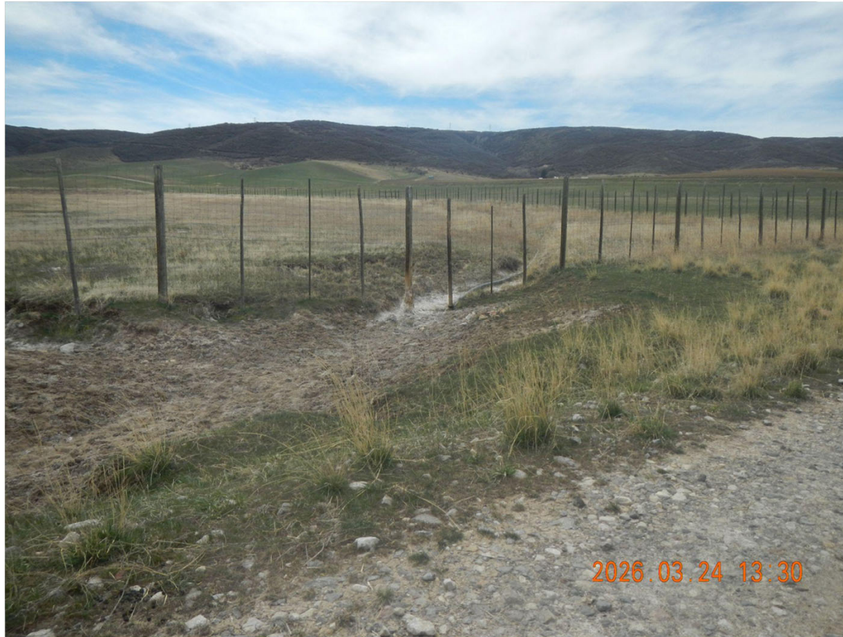
Photo 3– Culvert is diverting fluid from the fenced-in pit area north to the access road of the pit facility. Discharge point for facilities surface discharge permit is unknown. Viewing from the Northside of location looking South.
