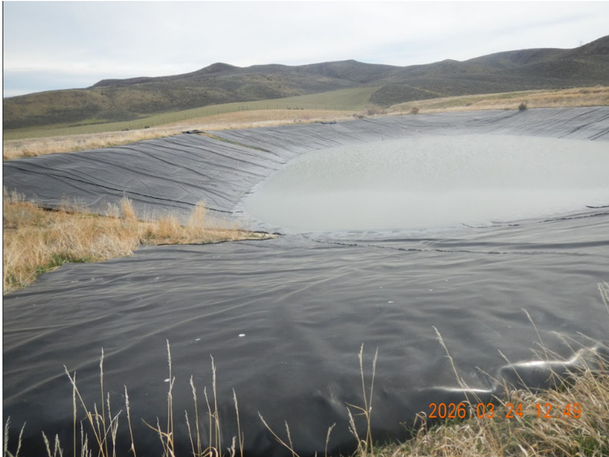
Photo 16 - Pit 4 looking west. Depth of fluids is approximately 12" to 24".
