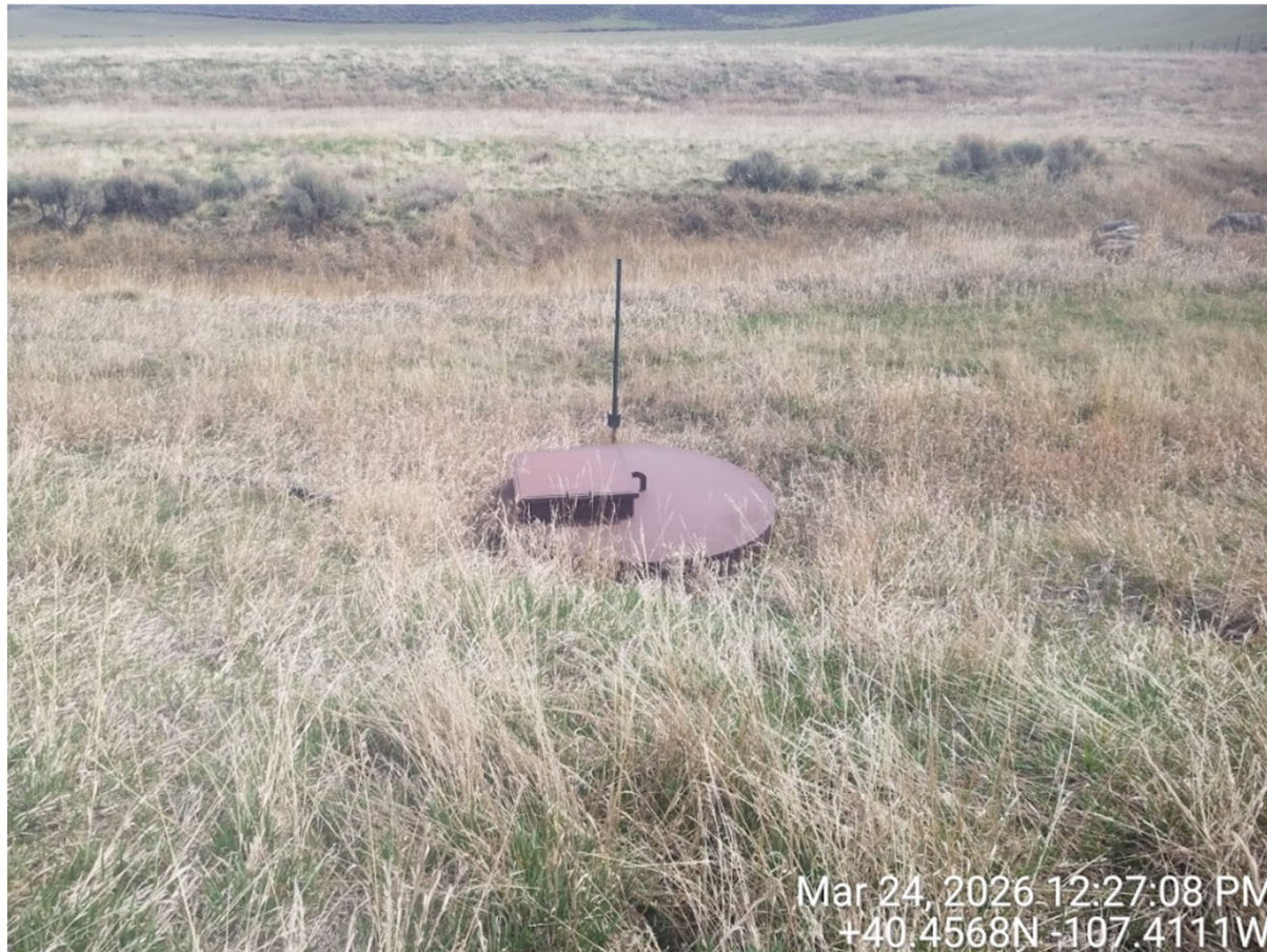
Photo 23 - Pit 7 valve can
