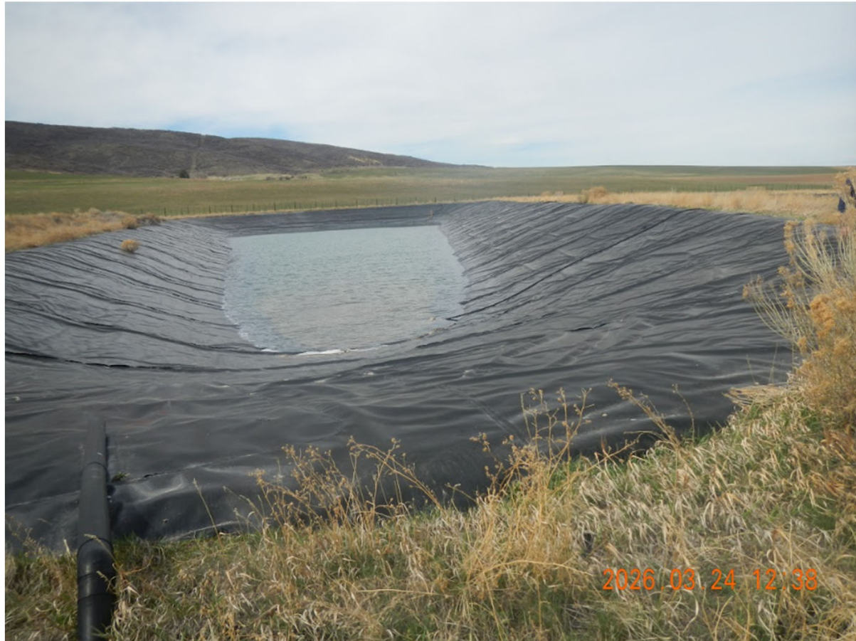
Photo 8 - Pit 2 looking west. Depth of fluids is approximately 12" to 24".
