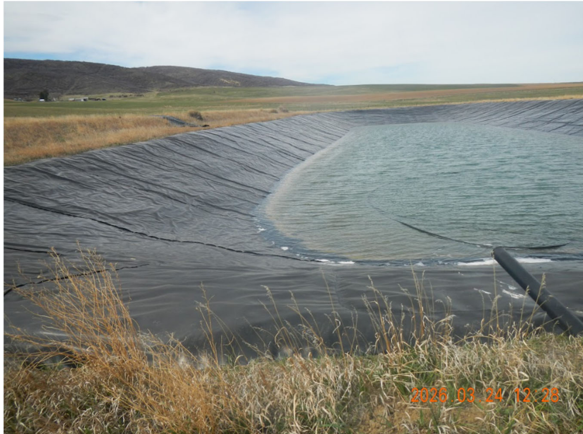
Photo 21 - Pit 6 looking West. Depth of fluids is approximately 12" to 24".
