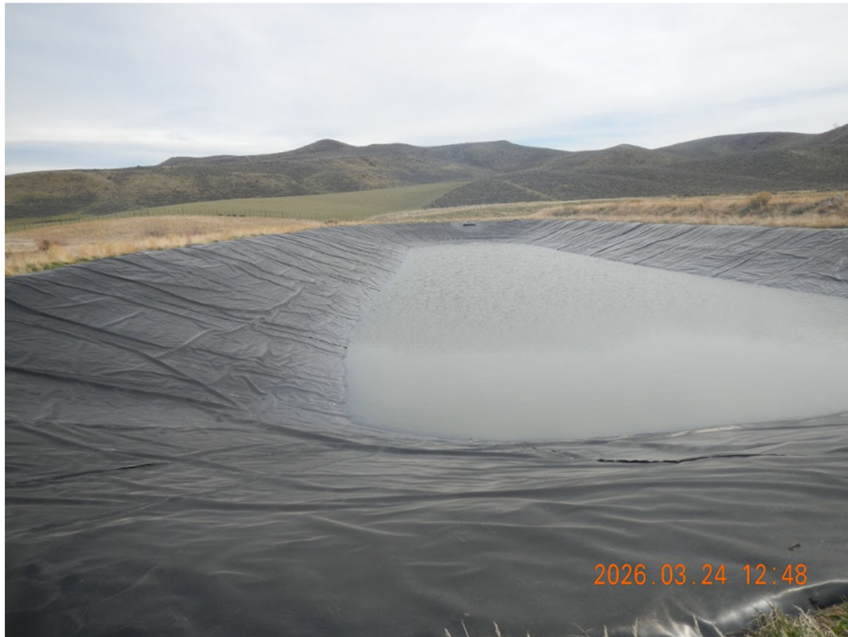
Photo 13 - Pit 3 looking east. Depth of fluids is approximately 12" to 24".
