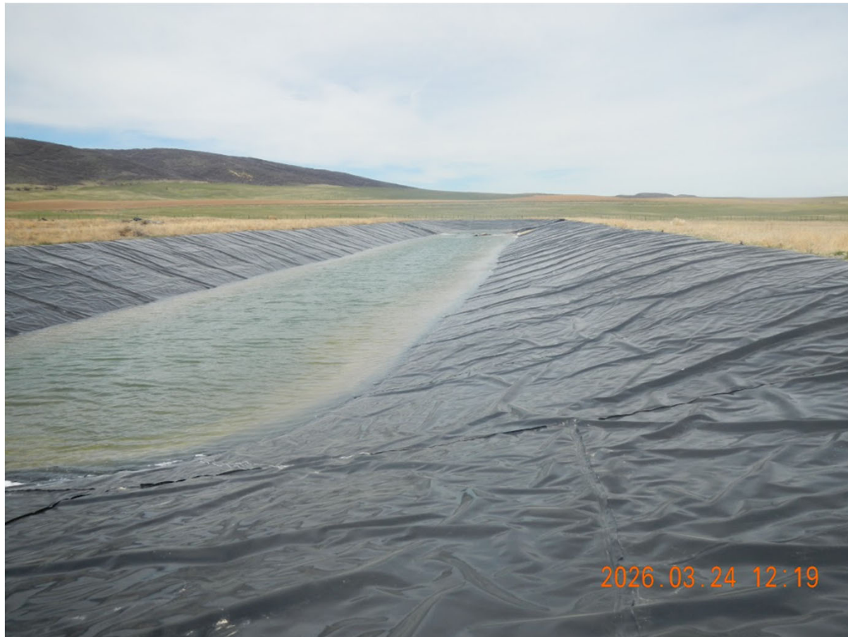
Photo 34 - Pit 10 looking West. Depth of fluids is approximately 12" to 24".
