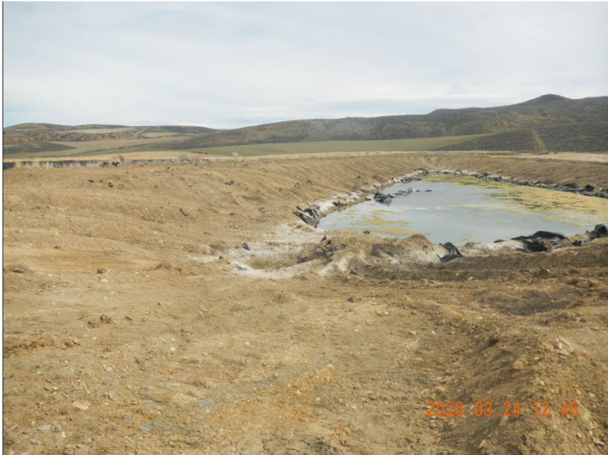
Photo 6 - Pit 1 looking east. Disturbance along the pit walls. Note that the majority of the liner has been removed with some liner remaining in the base of the pit.
