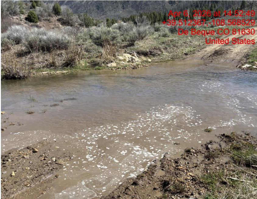
No BMPs or Erosion Controls at Stream Crossing – Photo #03415
