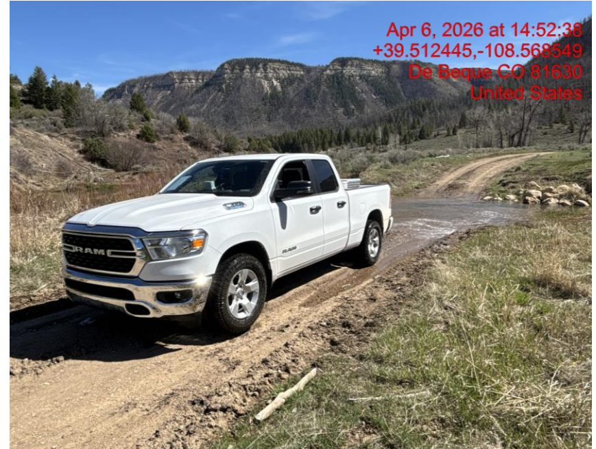
No BMPs or Erosion Controls at Stream Crossing – Photo #03414
