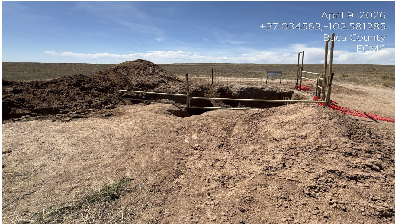
Photo 6. Facing west toward the excavated abandoned well site.
