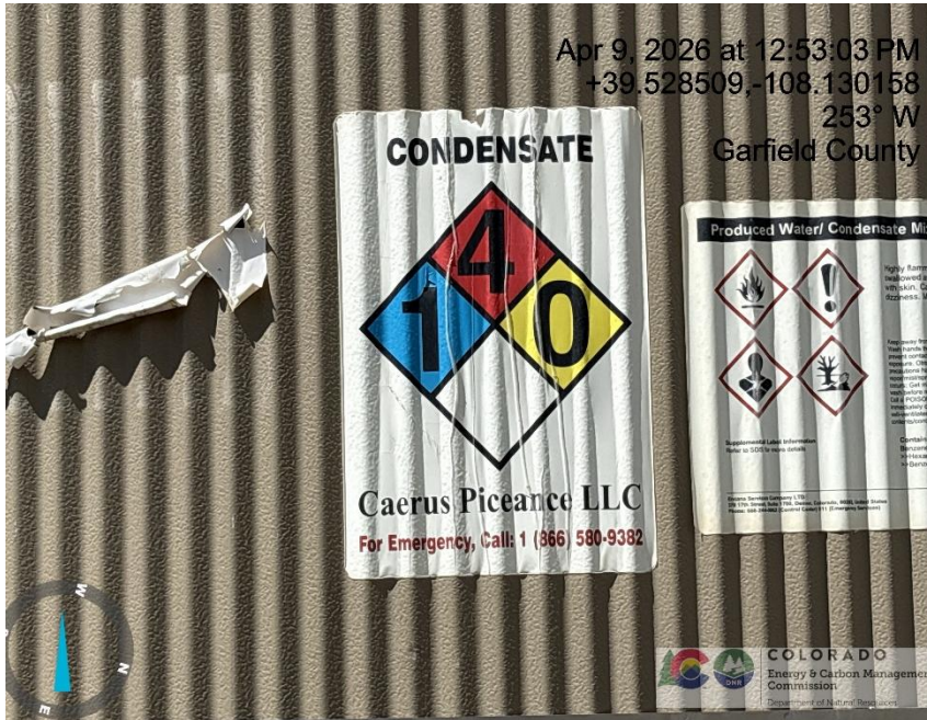
Photo # 6801 Tank label has previous operator name
