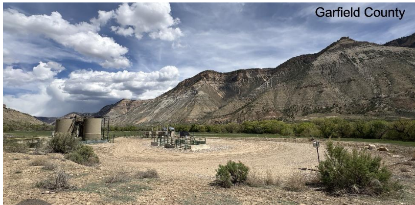
South West corner of location.
