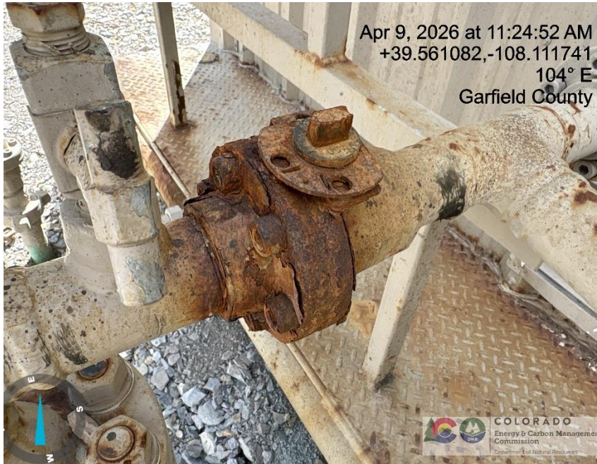
Photo # 6530 Mechanical Condition - Large amount of external corrosion visible on ball valve (N. PARACHUTE MF07C-4 C04 696 flowline)
