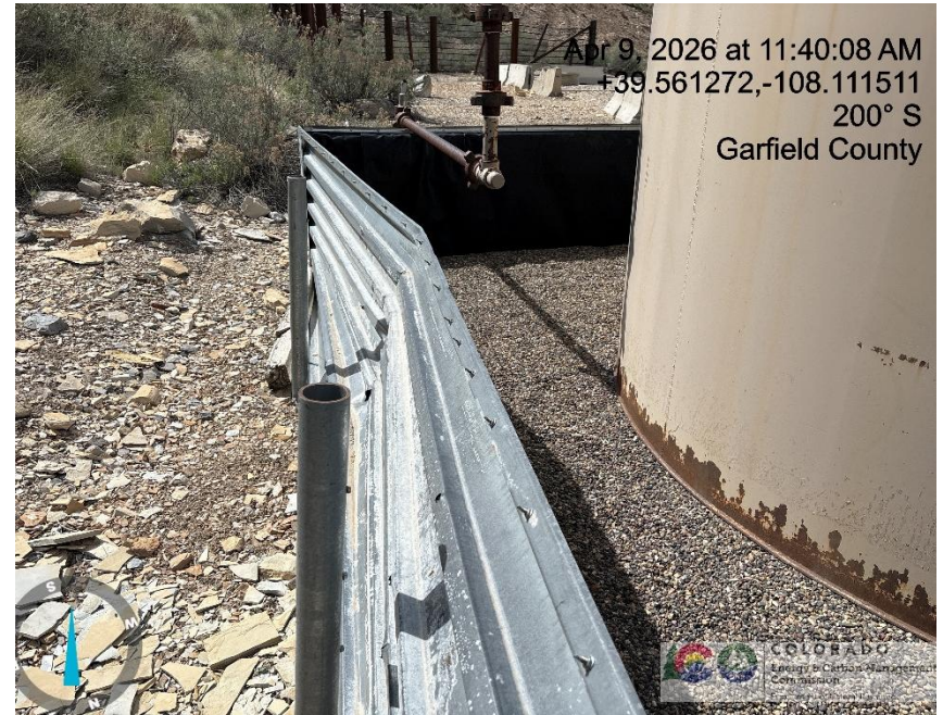
Photo # 6533 Damage to secondary containment
