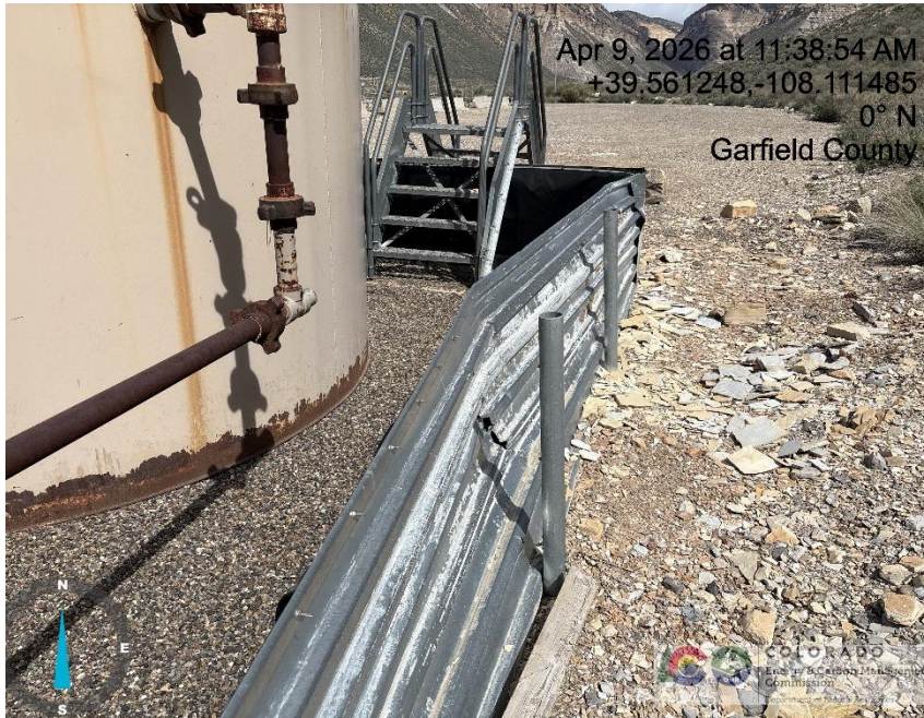
Photo # 6532 Damage to secondary containment
