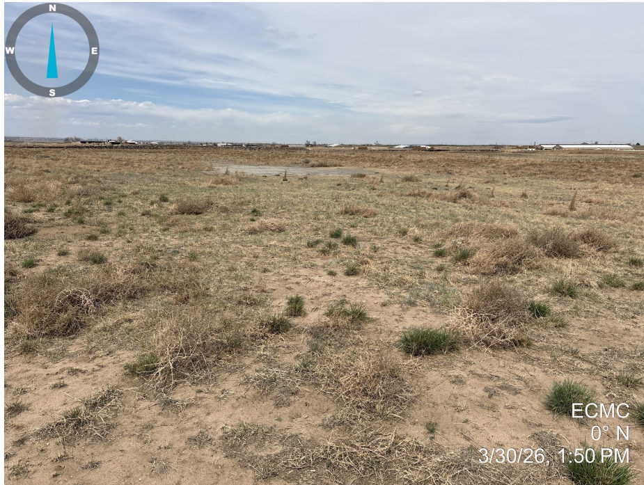
Photo 1. Photo taken of the well location, facing north. Photo illustrates that final reclamation activities appear to have taken place at the location, but vegetation establishment does not meet Rule 1004 standards. Weedy annual vegetation including russian thistle ( Salsola tragus ) was observed at the location.
