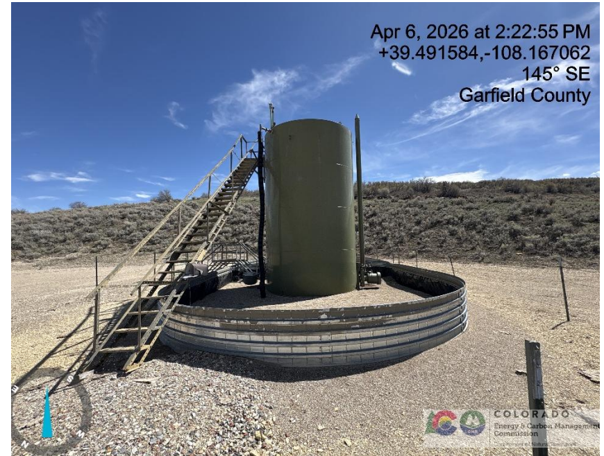
Photo # 5453 Tank battery lacks required signage
