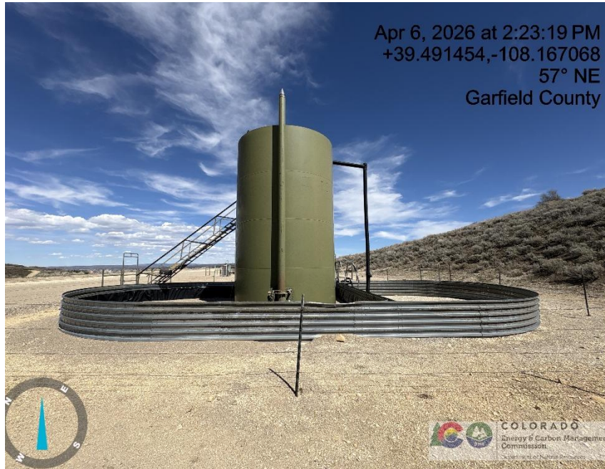
Photo # 5454 Tank battery lacks required signage
