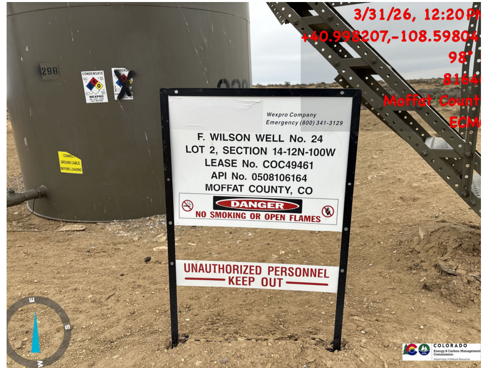
Battery signage lacks proper information
