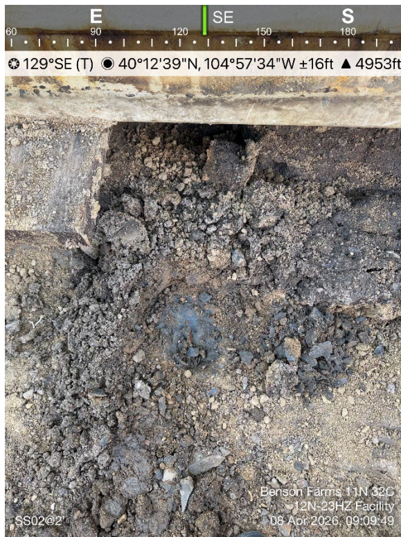
SS02@2' Screening Location
