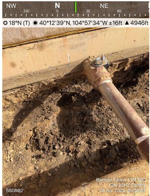
SS08@2' Screening Location
