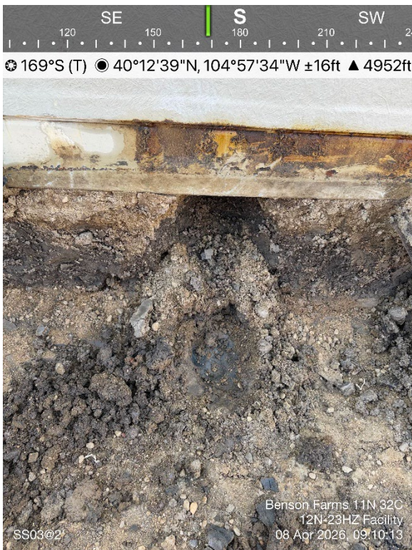
SS03@2' Screening Location
