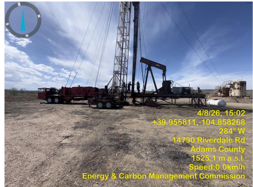
Photo 4 Well site, K.P.K. workover rig.
