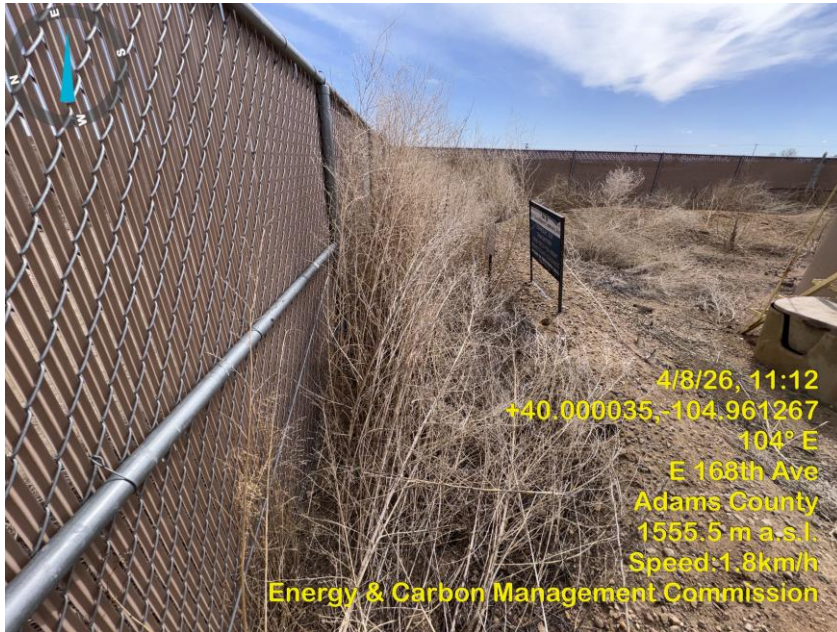
Photo 15 Dead vegetation/debris inside tank battery fencing.
