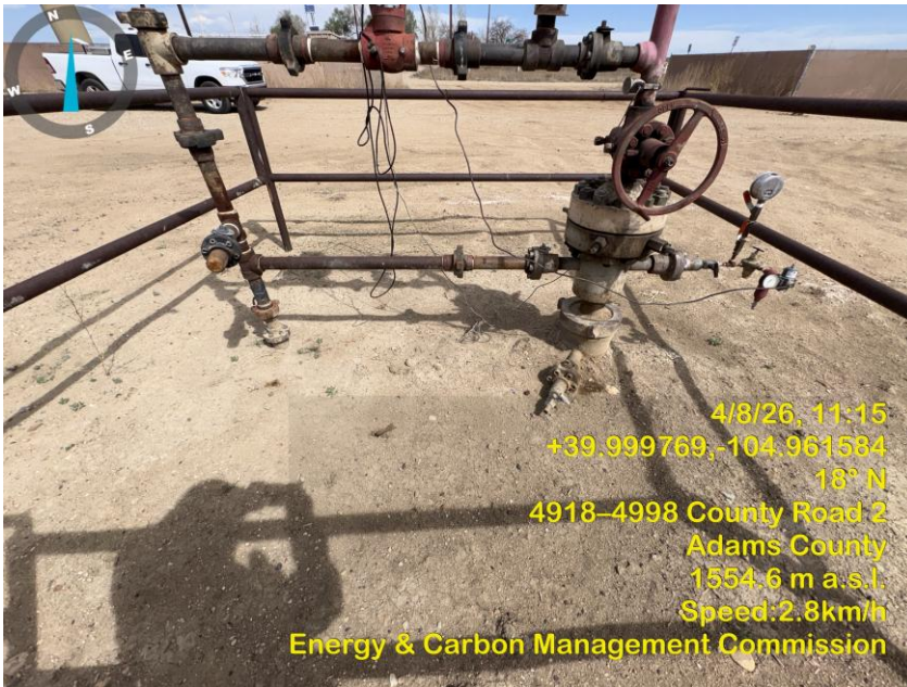
Photo 23 Stained soil by the bradenhead valve under the master valve.
