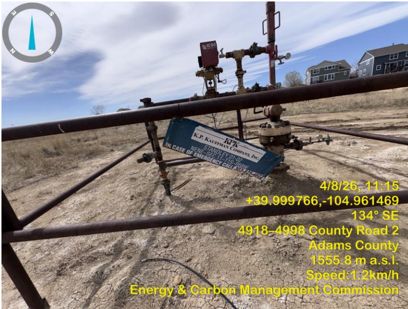
Photo 21 Wellhead sign needs to be secured to fence.
