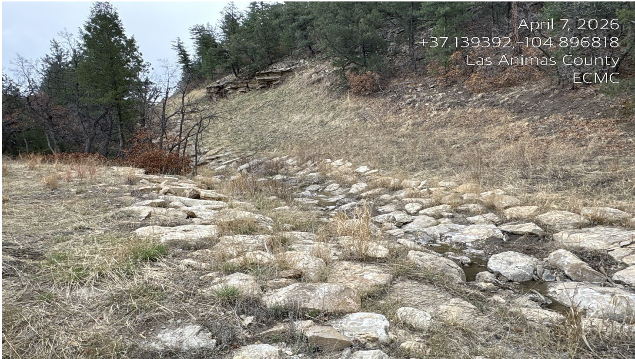
Photo 5. Facing northeast at the drainage crossing.
