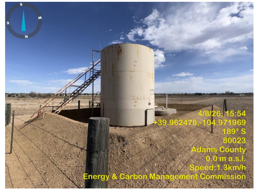
Photo 4 Tank battery.
