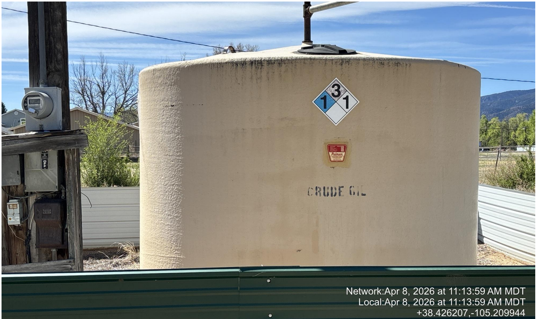
PHOTO 6: CAPACITY IS NOT POSTED AT CRUDE OIL TANK BATTERY. POST TANK CAPACITY AT TANK BATTERY, COMPLY WITH RULE 605. THIS IS A FOLLOW-UP TO INSP'S 695108710 AND 687903596 IMMEDIATE ACTION IS REQUIRED.
