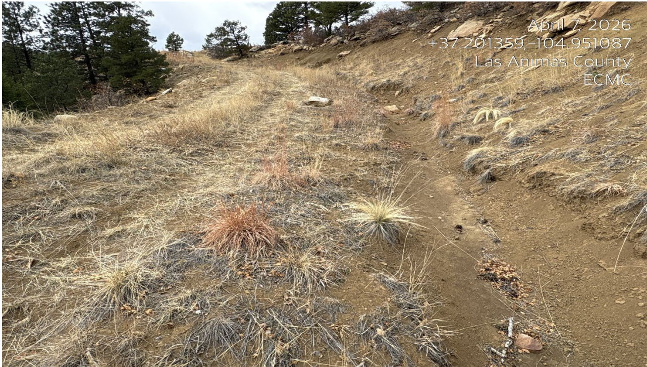
Photo 4. Facing west along the access road. Stormwater is directed down the length of the road side causing the erosion in the previous photo.
