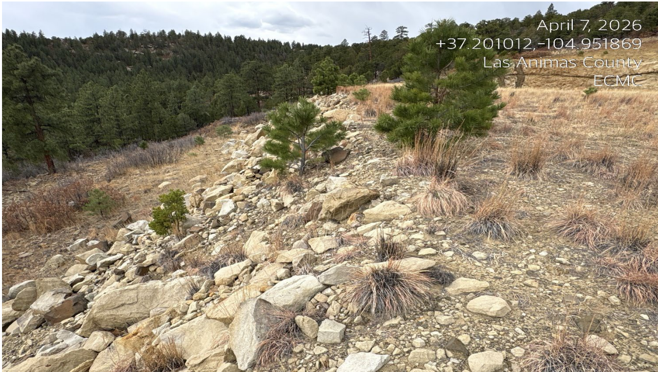
Photo 7. Facing west along the fill slope.
