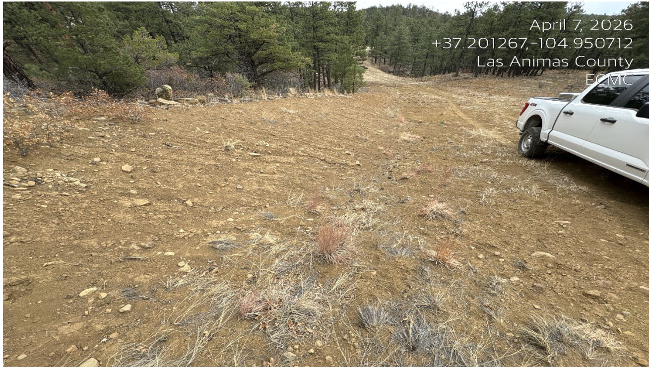
Photo 3. Facing east back down the road side. This area could use additional reseeding to establish vegetation.
