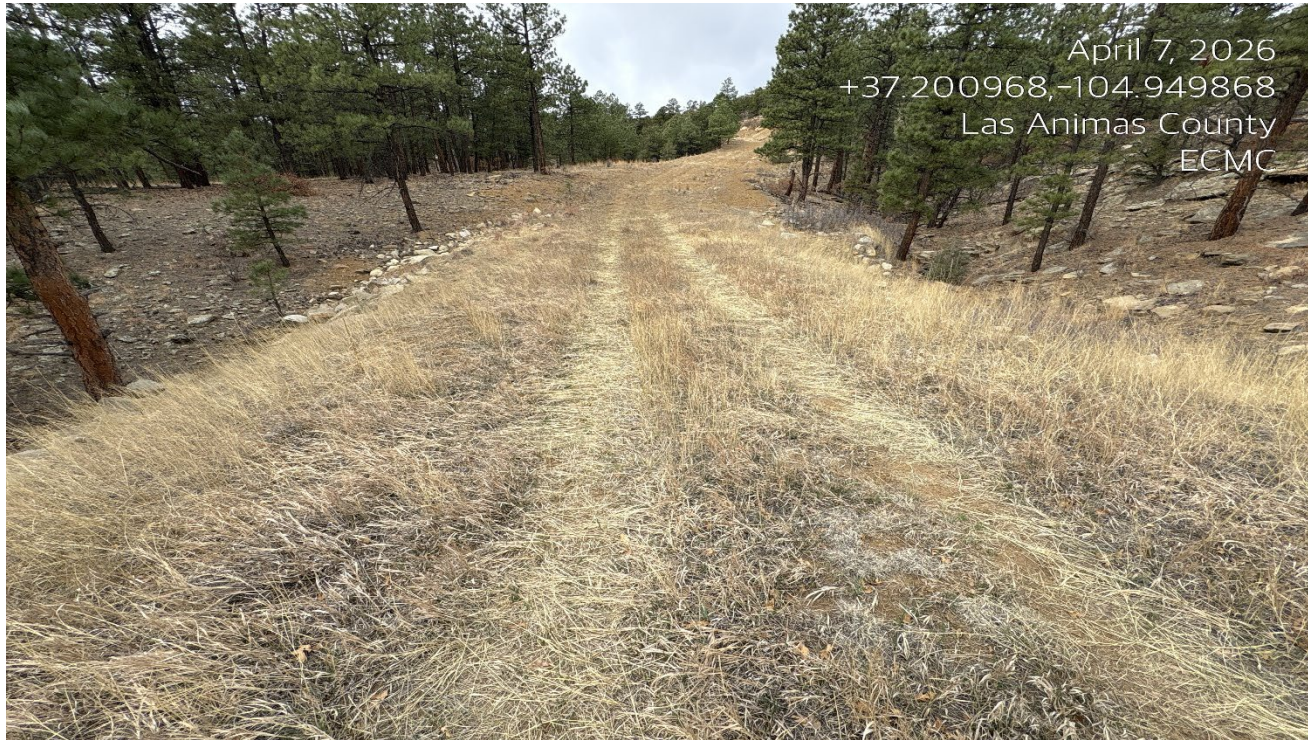
Photo 1. Facing west along the access road that remains per approved variance.
