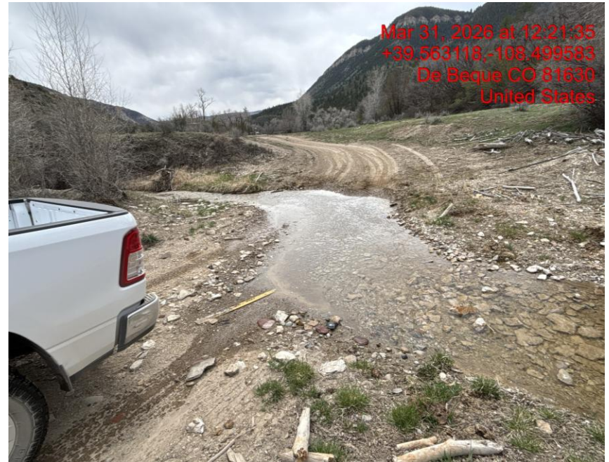
No Erosion Controls Installed at Stream Crossing – Photo #03366
