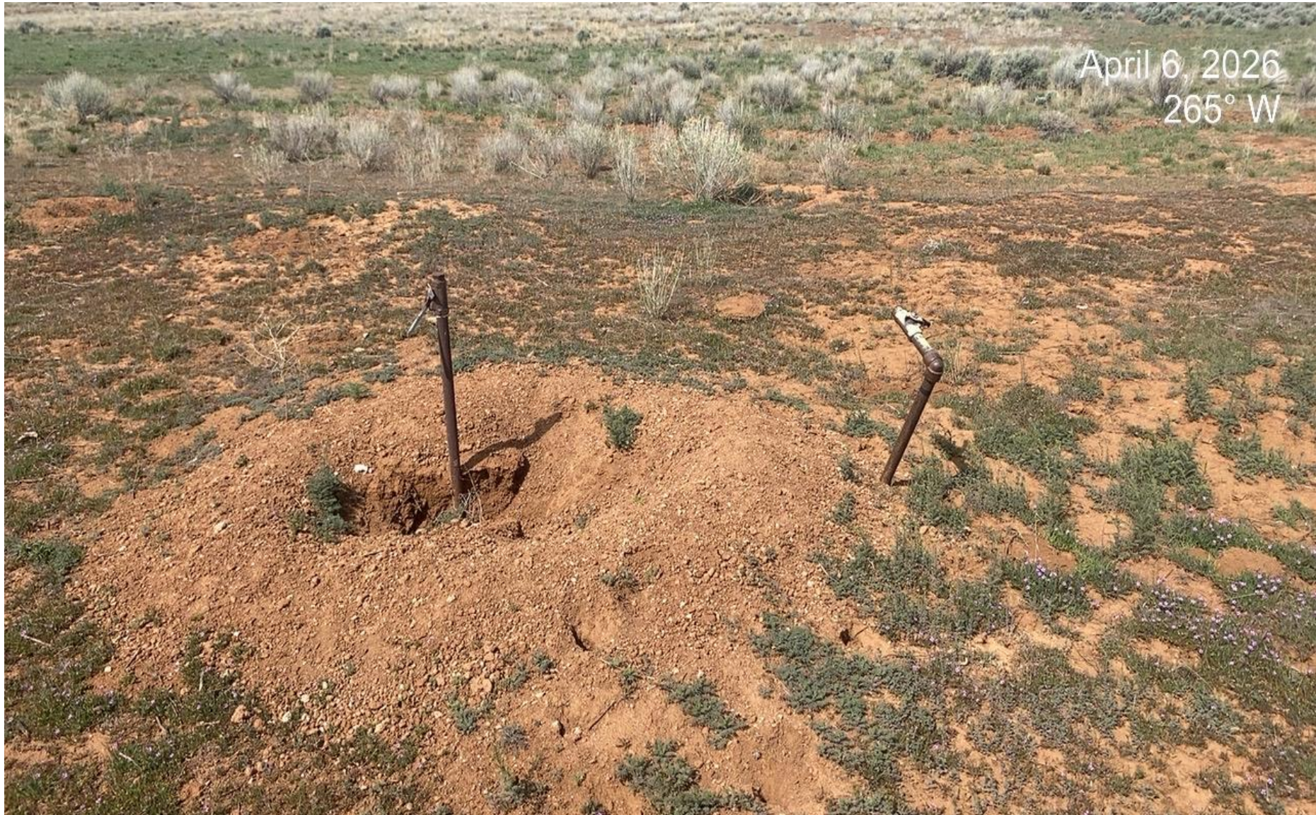
Photo 2. View of unused risers that remain on the western edge of the pad.
