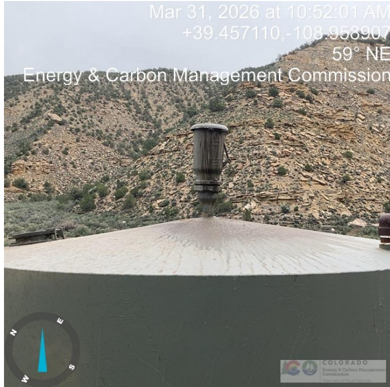
Staining on top of condensate tank and pressure relief valve.
