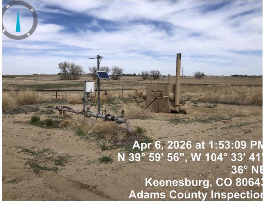
PHOTO#2 GAS METER/SEPARATOR
