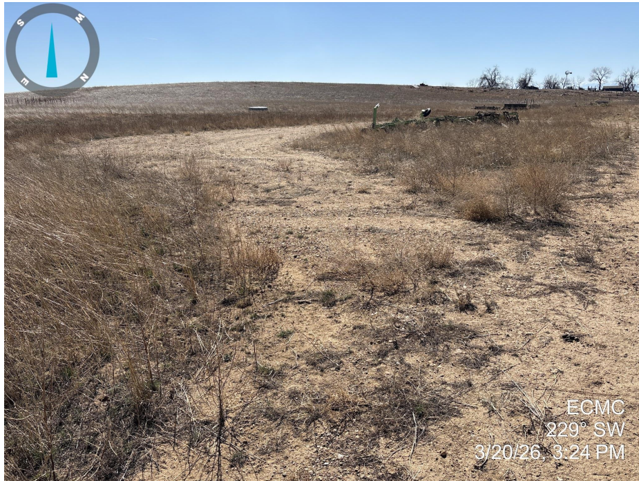
Photo 7. Photo taken of the tank battery location, facing southwest. Photo illustrates that final reclamation activities have not taken place along the access road and vegetation has not yet established to Rule 1004 standards.
