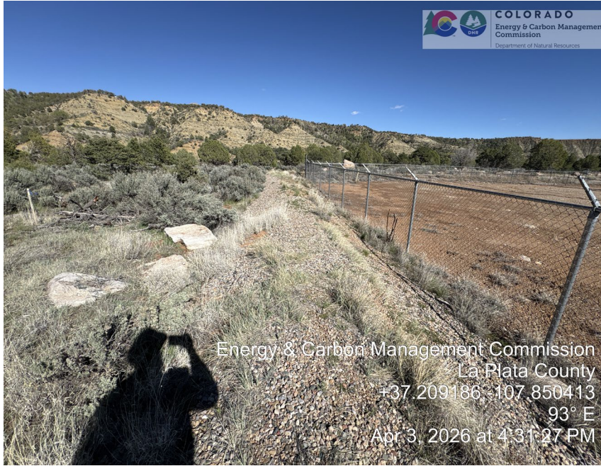
17. Location perimeter berm.
